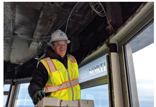
Using the SX10 in tight, enclosed spaces.
